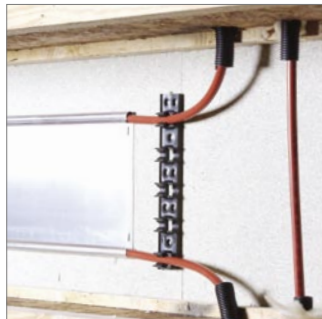
1 REHAU SOLUS System 400mm joist spacing
